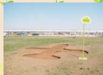
from construction site...
